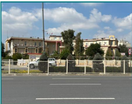
Serviceability(AC units, pipes, etc) Dishes/Antennas
