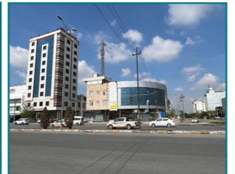
Cell tower - Wires
